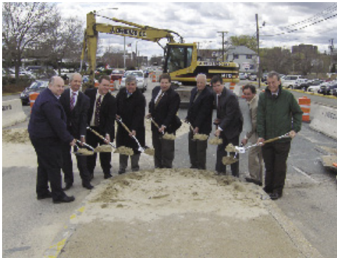
Shown are city officials at a May ground breaking ceremony to begin the underground utility work for the new urban boulevard.
